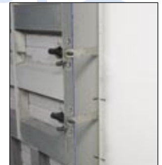
T-Stud with foam and nails
