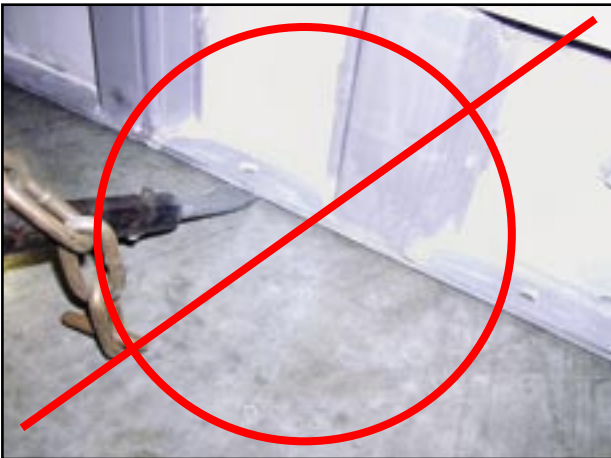
DO NOT insert the slip bar under an unsupported section of endrail.
