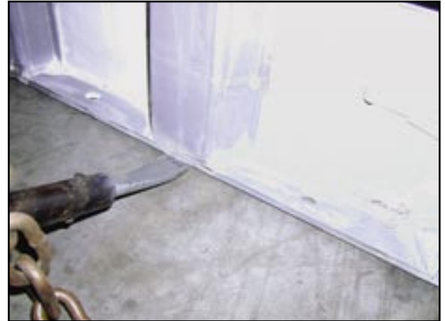
Place the slip bar under a section supported by a vertical brace.
